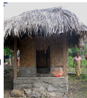
A Composting Toilet
