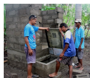
Local builders building a toilet
