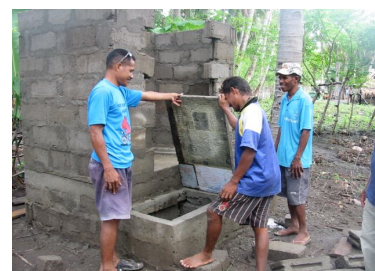
Building a Composting Toilet on Atauro Island
